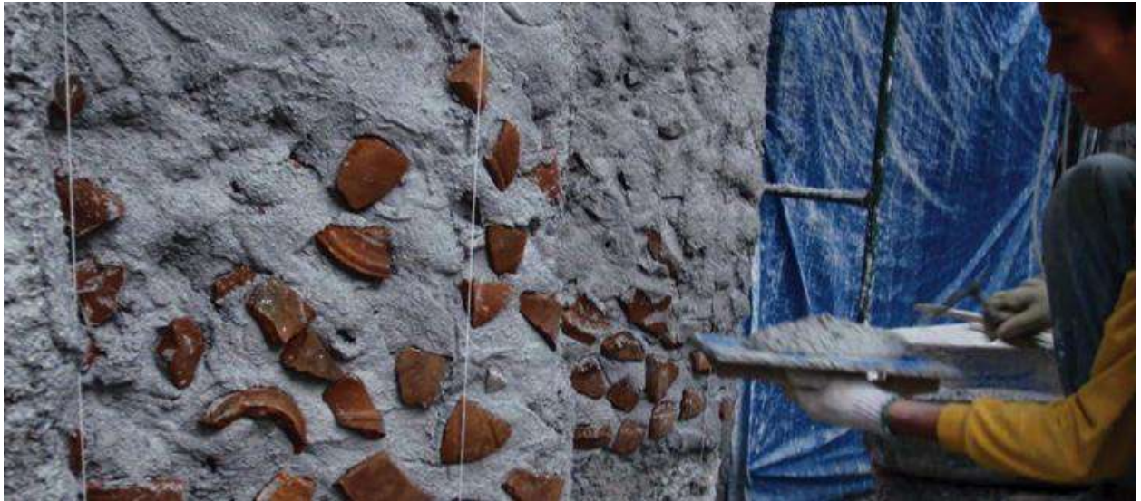
Figure 2: Infill of Lost Volumes
