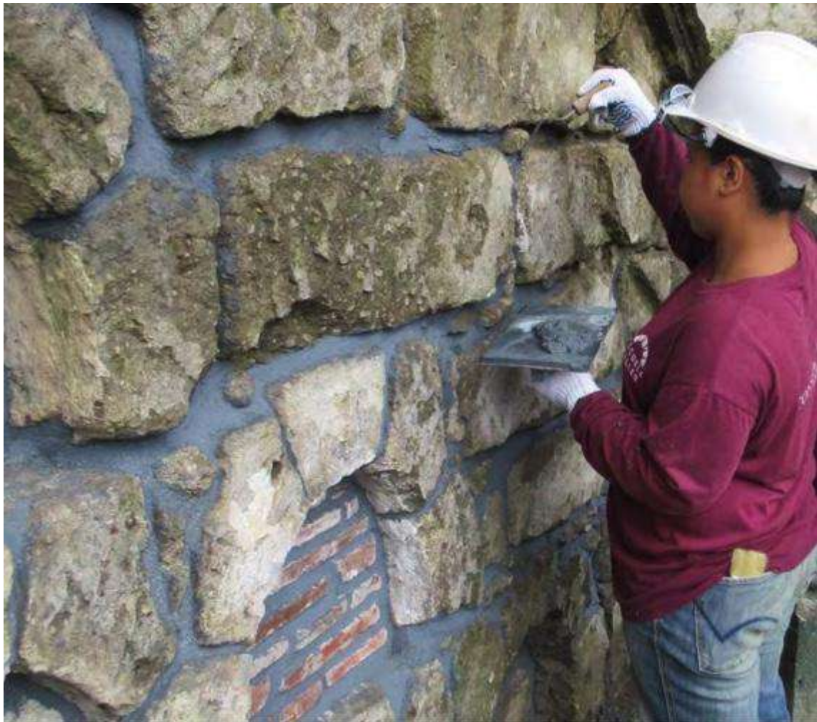
Figure 3: Repointing in Process
