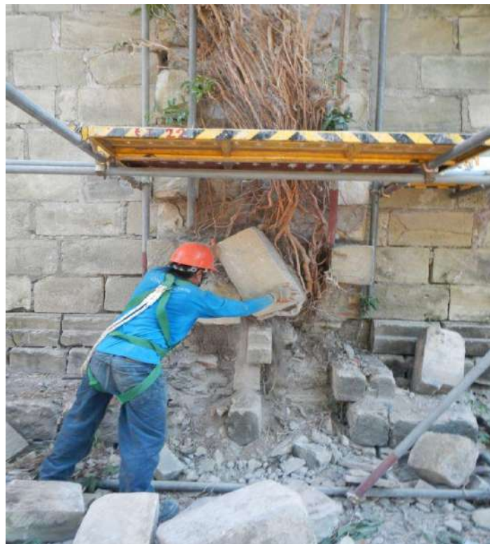
Figure 6: Disassembly of Stones
