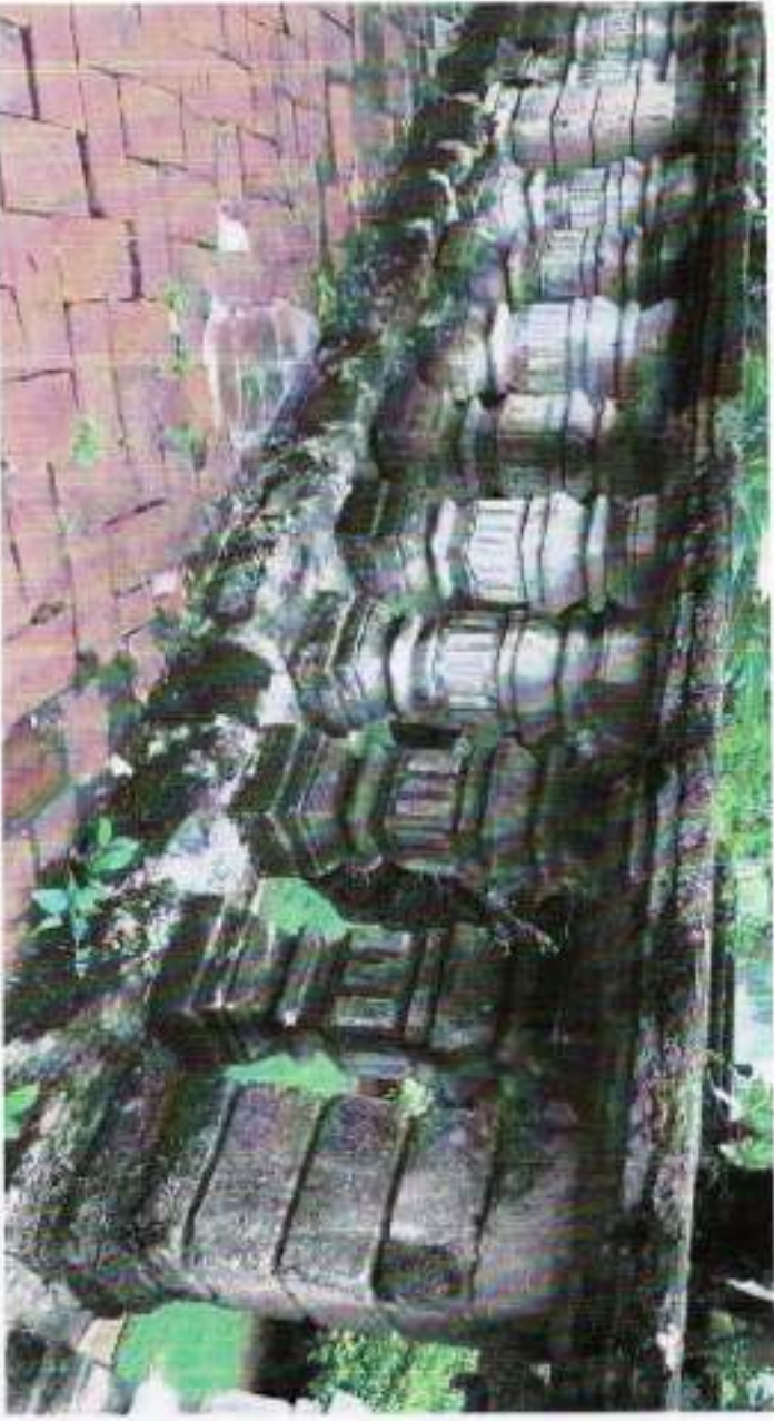
BALUSTRADE 15 (Left Side facing Chapel)
