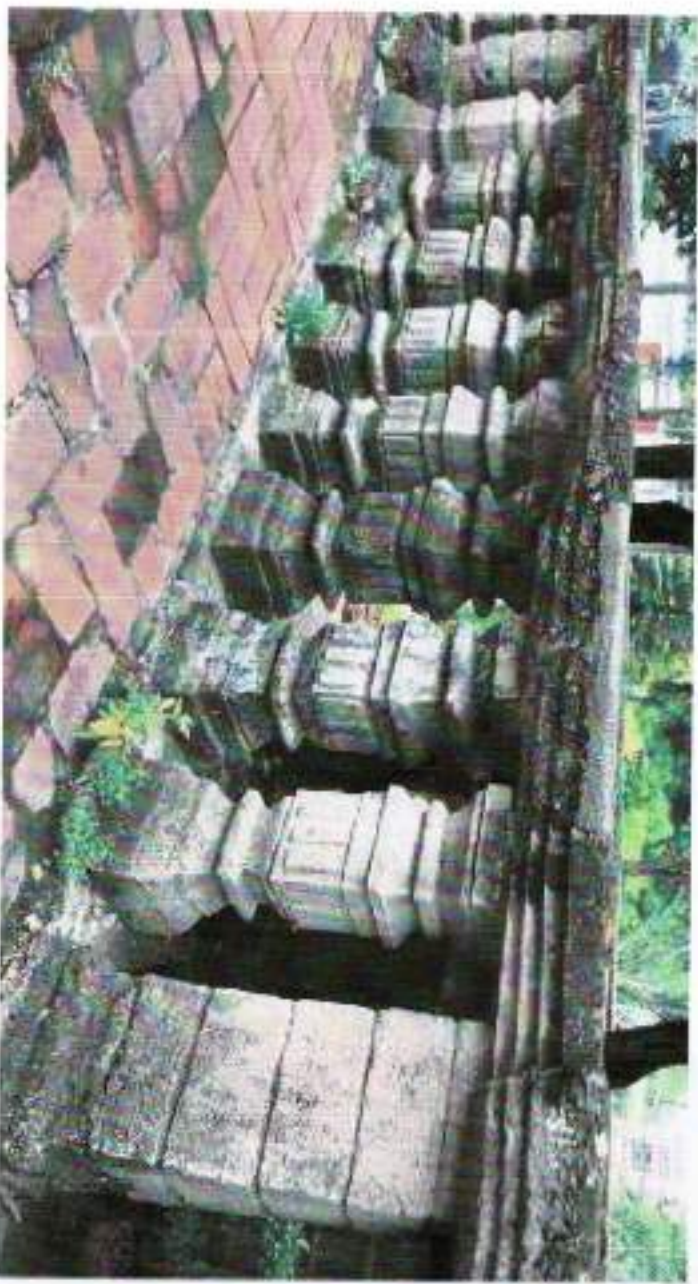
BALUSTRADE 28 (Left Side facing Chapel)
