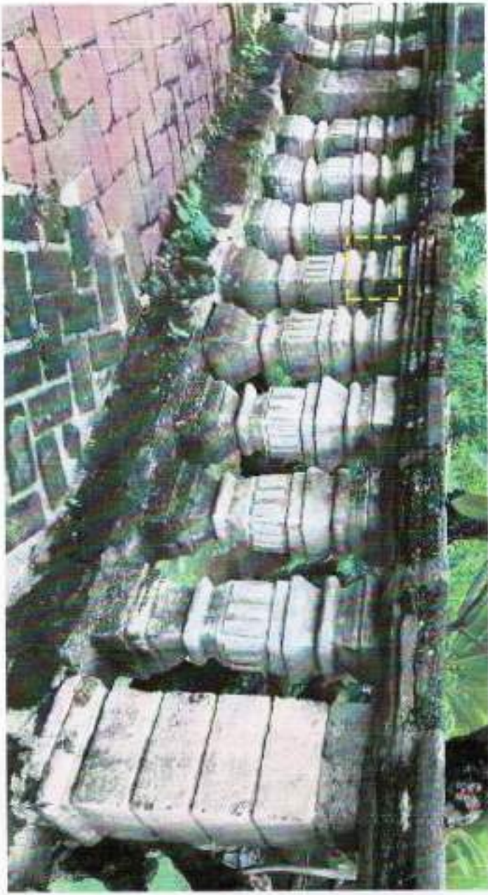
BALUSTRADE 16 (Left Side facing Chapel)
